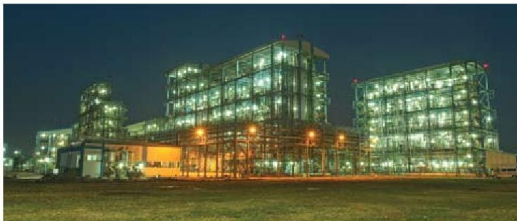
A MAJOR PRODUCTION HUB: The Dahej complex started up in 2012 and is now SRF's largest manufacturing site. The company uses only 40% of the land available there.
