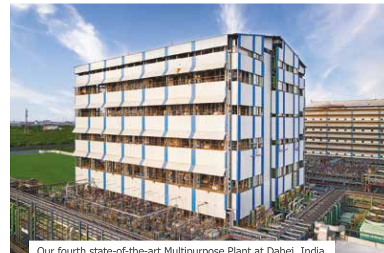
Our fourth state-of-the-art Multipurpose Plant at Dahej, India
